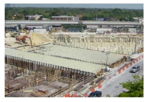
several sections reduced the concrete pour for the bottom slab into manageable sizes.
